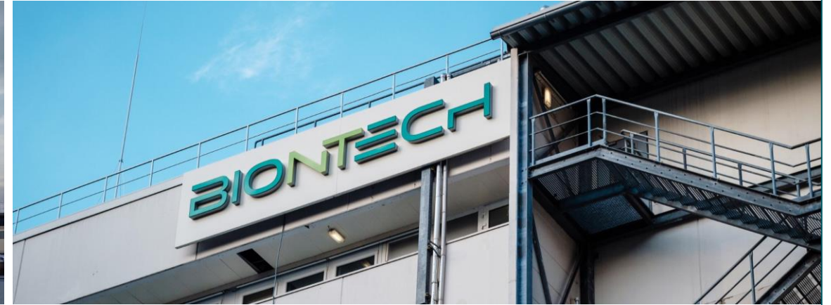
Bulk mRNA production facility, Marburg, Germany
