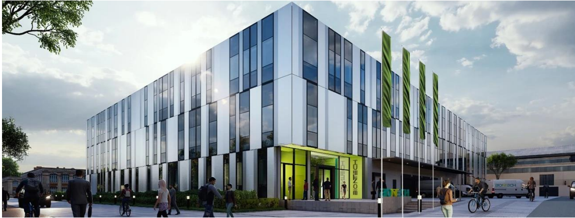
Personalized mRNA production facility, Mainz, Germany
